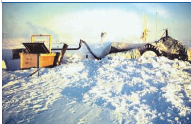
To help start the tractor, it was parked under a tarp near the buried generator shed. The exhaust of the diesel electric generators was piped up under the tractor to aid in its starting.
