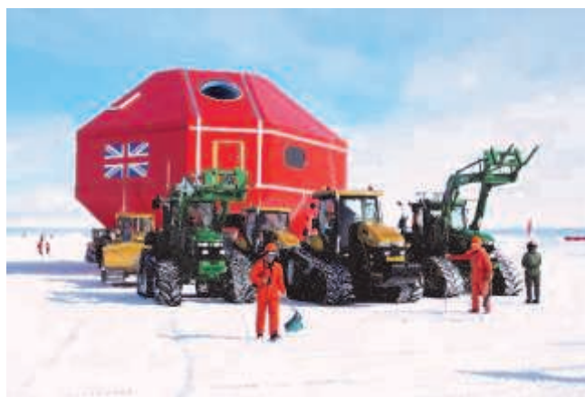
Moving "A" module. In 2011, fifty five years after the original Halley Base Hut was built, the 200 ton module was on skies and was pushed and pulled out of a seven-foot deep bulldozed ramp by two John Deere tractors, two Cat Challengers, and four D4 or D5 Cat Dozers. Once level with the snow, the module was completed, and the John Deere's and Challengers moved the module over 9 miles in two hours to the new Halley VI location. Credit Halley Bay VI party.
