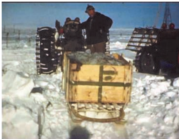
Here the tractor's winch is being used to bring ice and snow up the ramp from the door of the generator shed, which was buried 30 feet below the surface.
