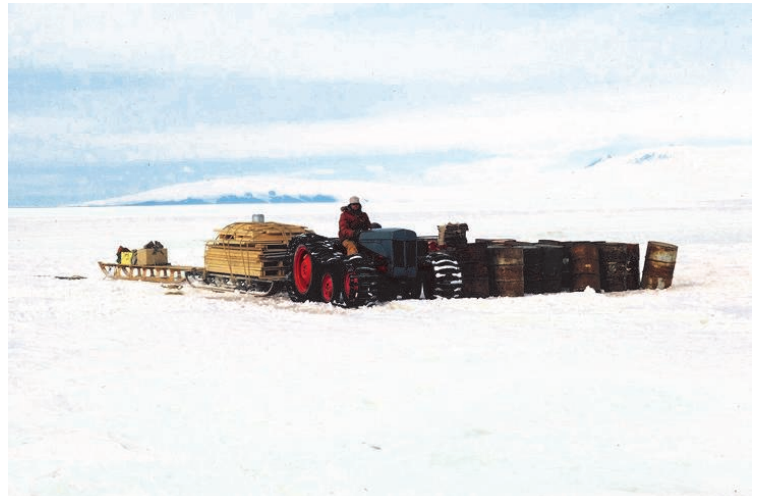
4. Derek Cordes at the TEA20 about to leave the Bay of Sails for a crossing of the Wilson Piedmont Glacier. The sledge is loaded with building materials for a refuge hut near the shore of Lake Brownworth at the foot of the Wright Lower Glacier in the Wright Dry Valley. The return trip took more than six hours. (Nov 1968)
