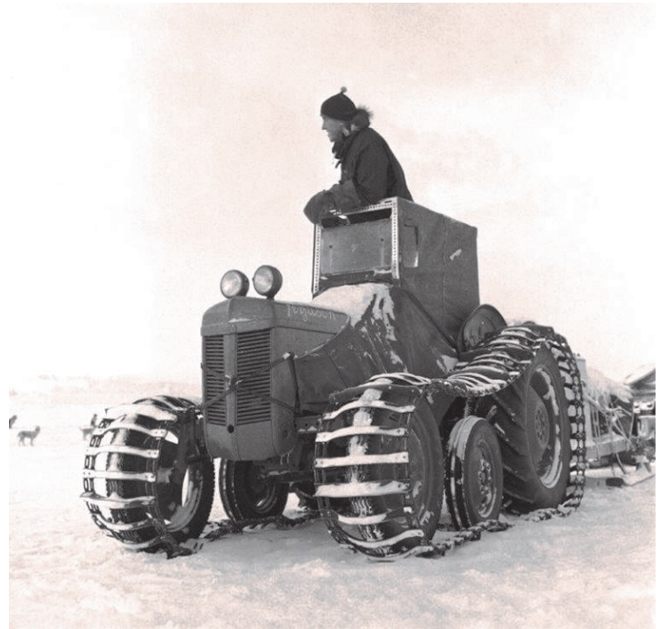
Tractors bound for Cape Crozier with Sir Edmund Hillary on top. You will notice the better canvas cab. If you look closely you can see the extra brace for the front axle. The tracks are still made of chain links. The frame of the front of the cab was made out of dexion shelving that they had on hand. Photo credit Transantarctic Expedition Images' Antarctica New Zealand. TAE #789
