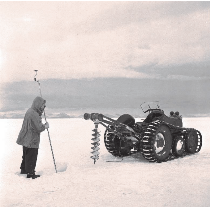
Miller testing depth of the sea ice with a Ferguson D-FE-20 Post Hole Digger. Photo credit Transantarctic Expedition Images' Antarctica New Zealand # TAE 693
