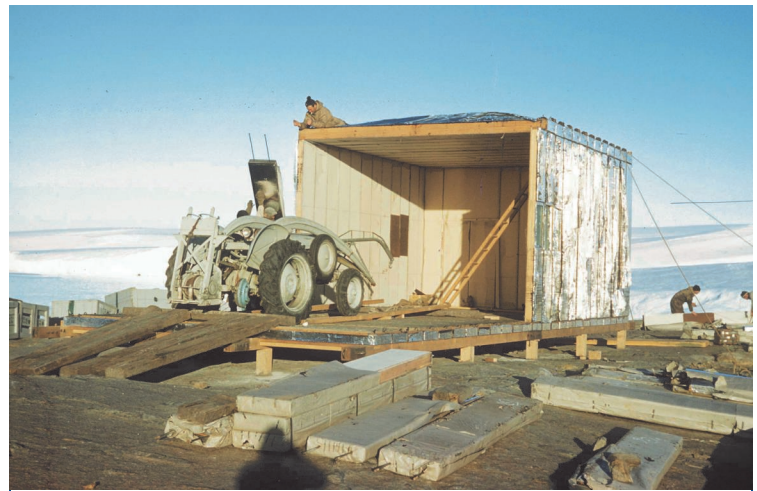
3978D3 Erecting Cosray hut, Mawson, February 1955
