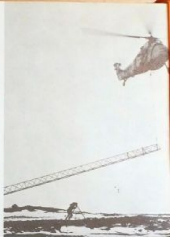
Helicopter helps raise a 110-foot rhombic communications tower.
