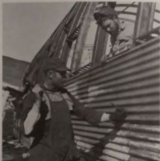
Carl E. Churchwell, SW1, puts up metal siding on a new hangar. Assisting him is Carl Hinson, SWE2.
