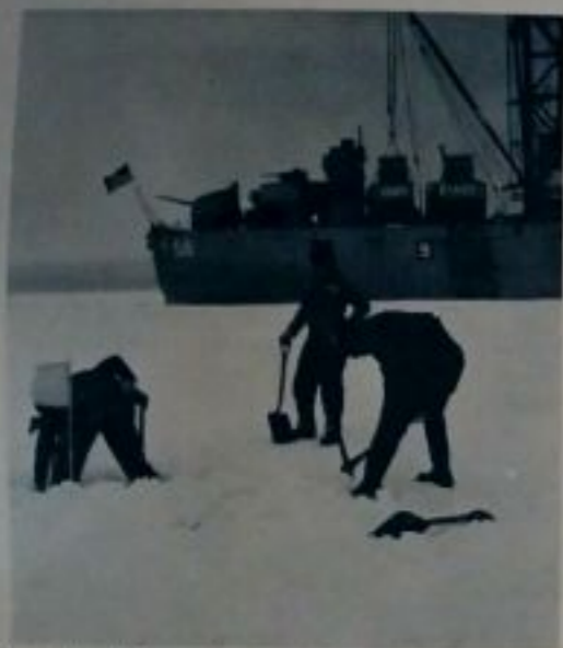
Deck hands from the Arneb chop holes in the ice for the "dead men," buried timbers, to which the ship will secure her lines.
