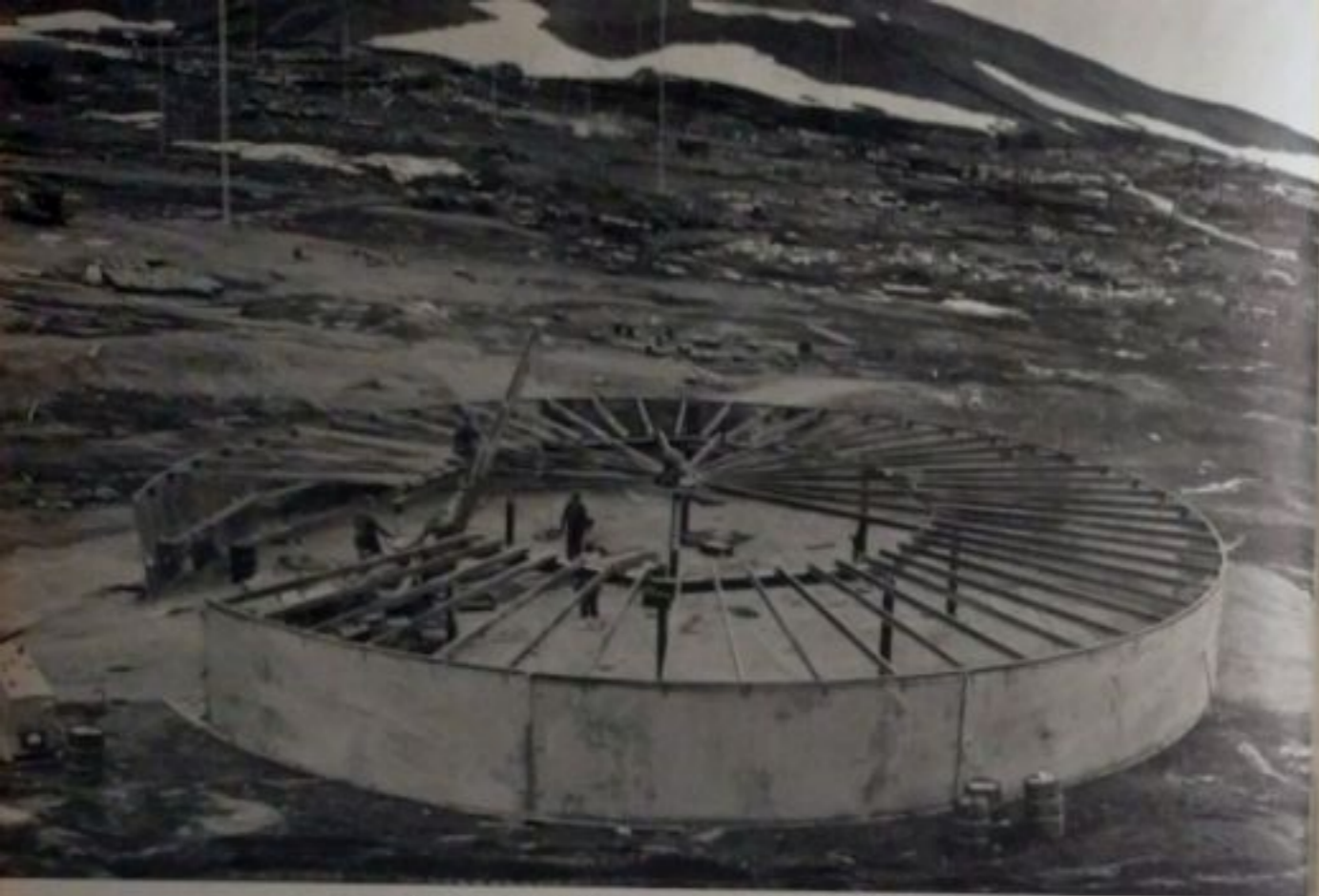
A new 250,000 gallon fuel tank being constructed at NAF McMurdo Sound.
