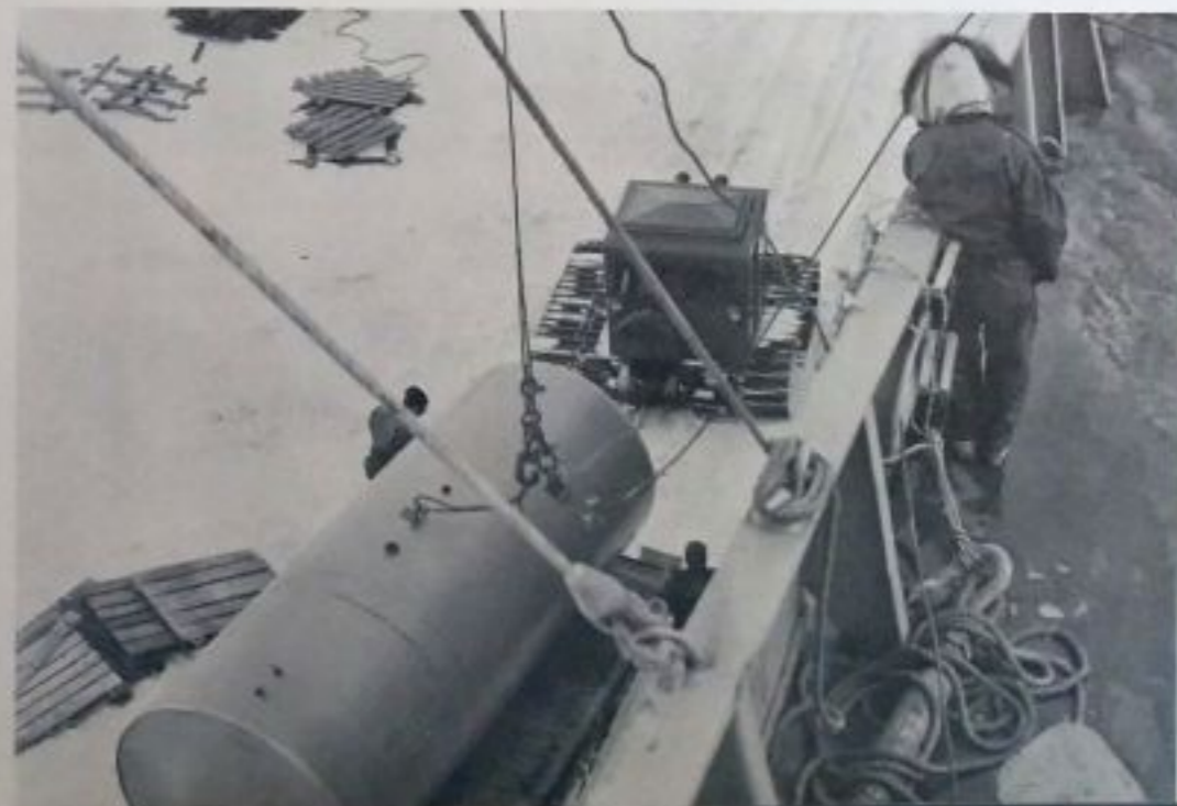
A standby generator is unloaded for the McMurdo camp.
