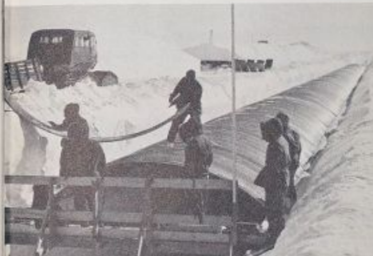
The arched roof creates a snow tunnel. For wider work a special construction bridge is used. The finished work will contain buildings. Improvement over "old" Byrd Station tunnel is apparent.
