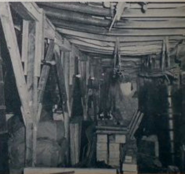
The arched roof creates a snow tunnel. For wider work a special construction bridge is used. The finished work will contain buildings. Improvement over "old" Byrd Station tunnel is apparent.
