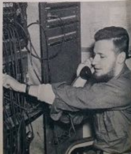
Stephen L. Kostielney, PN3, operating switchboard at NAF McMurdo Sound.
