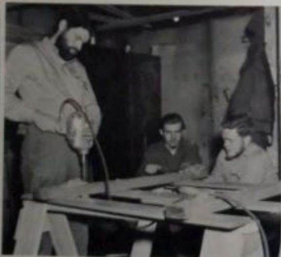
Robert D. Brown, BUL3, Raymond L. Smith, CN, and David R. Snyder, CN, repair a tail gate of a twenty ton sled.
