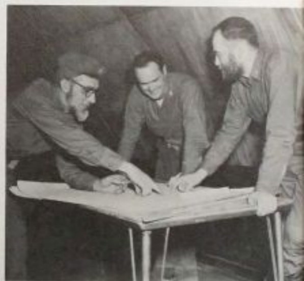
Archie E. Johnson, BUC, Lt Horace B. Jones and Lt Charles W. Gates plan construction of McMurdo Bowling Alley.
