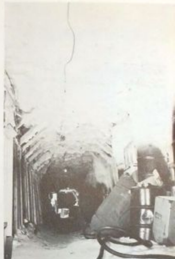
The men at Pole station live beneath 10-15 ft. of ice and snow. Each compartment is connected by one or more tunnels.
