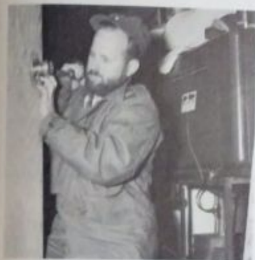
Jerry Bogle, BUL1, repairs a door handle in shop area.
