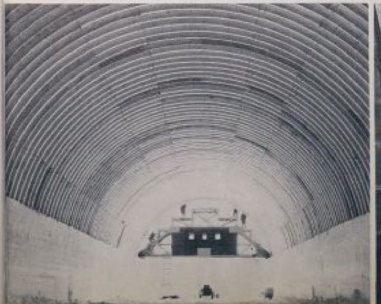
The arched roof creates a snow tunnel. For wider work a special construction bridge is used. The finished work will contain buildings. Improvement over "old" Byrd Station tunnel is apparent.
