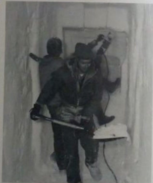
Right: Ronald J. Poniewaz, BUR3, and Robert J. Niedermayer, BUL3, open one of the passageways which connect the large tunnels.
