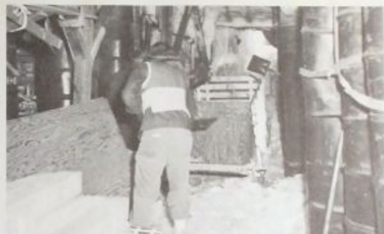
Ice and snow accumulations are removed from the tunnels with the use of sleds.
