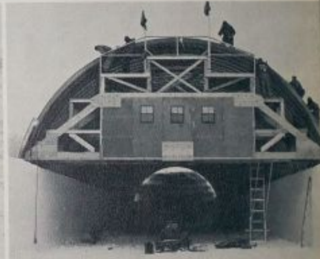
The arched roof creates a snow tunnel. For wider work a special construction bridge is used. The finished work will contain buildings. Improvement over "old" Byrd Station tunnel is apparent.
