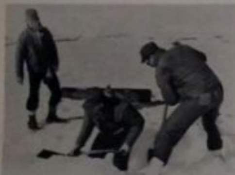
Ballew, SN; Bowman, SN, and Wright, SN, dig hole for placing a "deadman."
