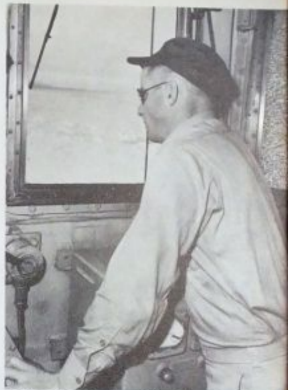
In the aloft conning tower 90 feet above the waterline, Glacier OODs control both rudder and engines as the icebreaker rams her way through the pack.
