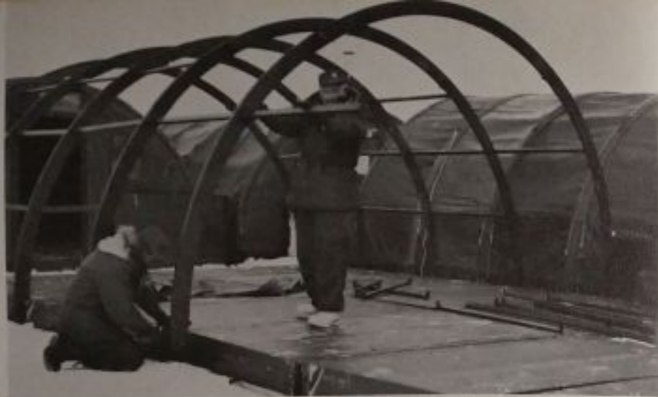
The men at Williams Field live in Jamesway type huts shown here during construction.
