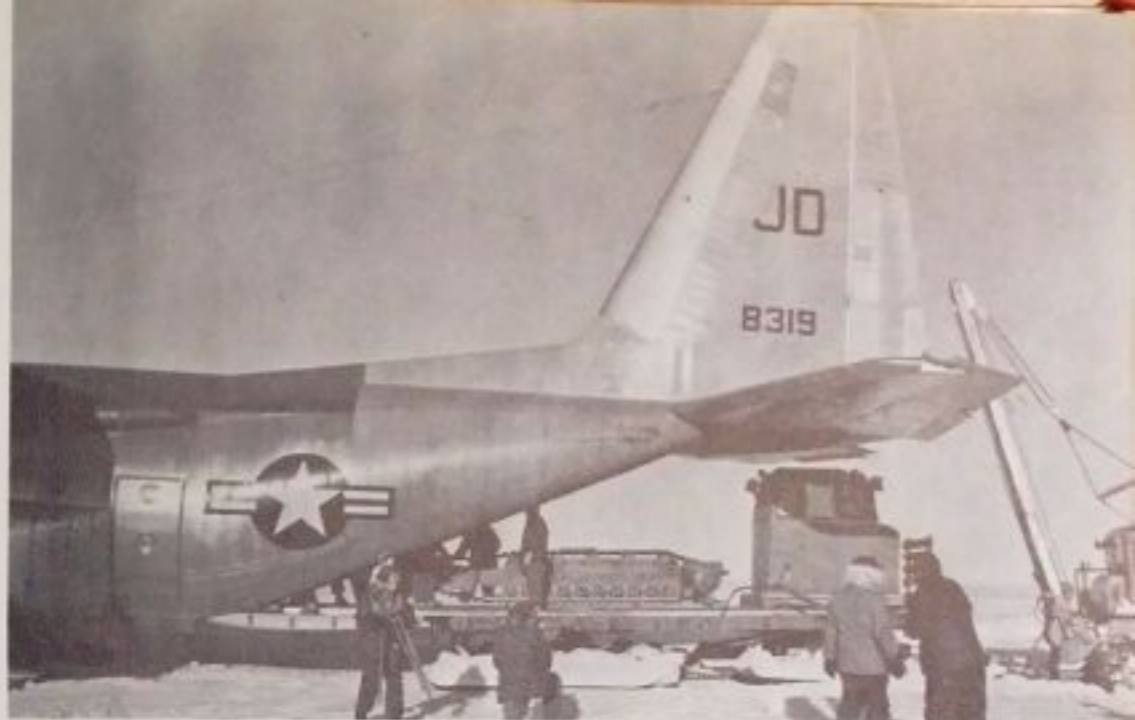
C-130 digests parts of Peter Snow Miller for transportation to new Byrd Station site.
