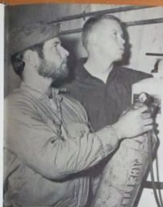
Charles T. Jones, UTP2, and Darrel Gregory, UTCN, repair water heater.
