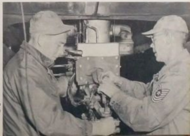
Sergeants Wade Howe and John Lindstrom make a last minute inspection of landing gear before the long flight to McMurdo.
