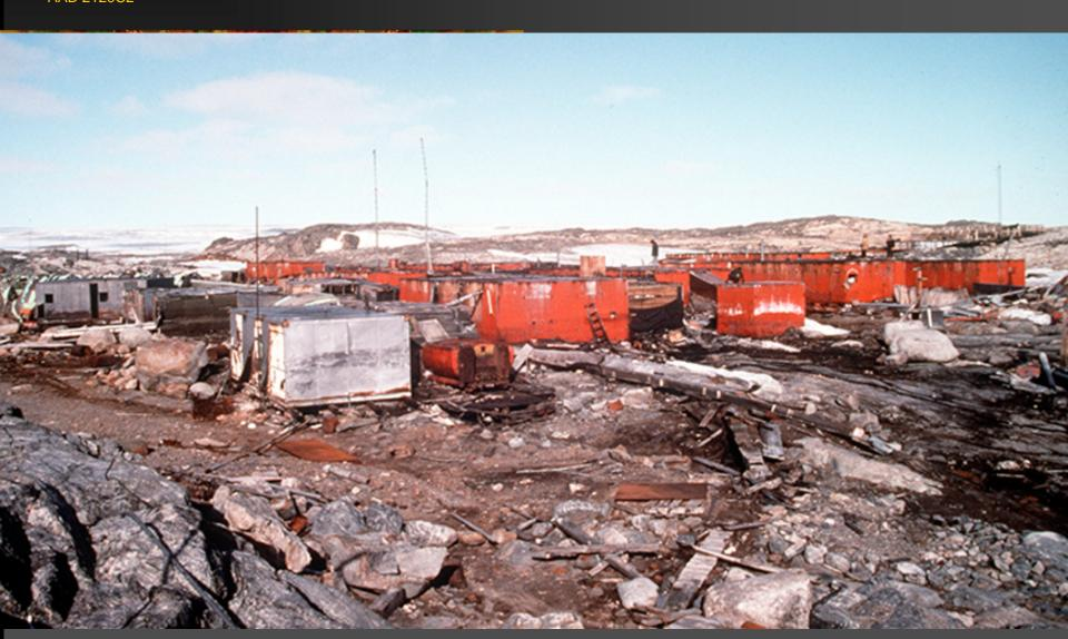
Keeping buildings maintained and intact allows for their future interpretation and visitor access. Triple glassed window hatches in the roof panels have been broken and as a result the interior of the building has filled with drift. Photographer R.Reeve Copyright AAD 2118B2
