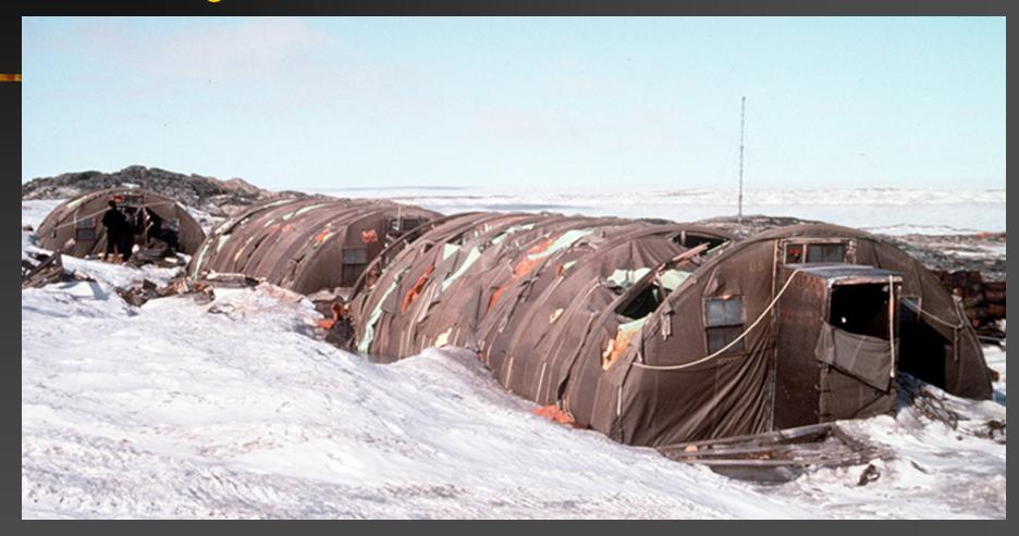
Later these buildings housed stores. While these photos were taken in 1992 even less of these double thickness canvas structures with fibreglass insulation remains in 2001.
